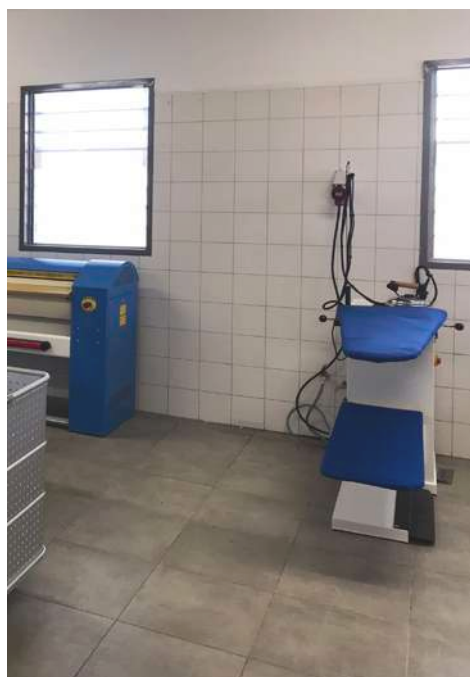
Laundry room inside several district hospitals in Ghana (Buipe, Somanya, Sawla, Tolon, Wheta and Bamboi)
